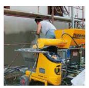
Easy to use Fed by an automatic mixer (Turbomix M22) for readymixed plasters in bags, it is easily run by a single operator who can regulate the material flow directly from the application point.
